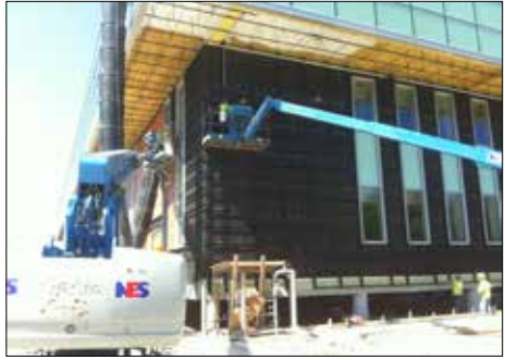
Vertical rails are attached to clips welded to the building's steel girders.
